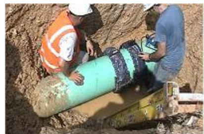
Guidedwave Ultrasonic Inspection
